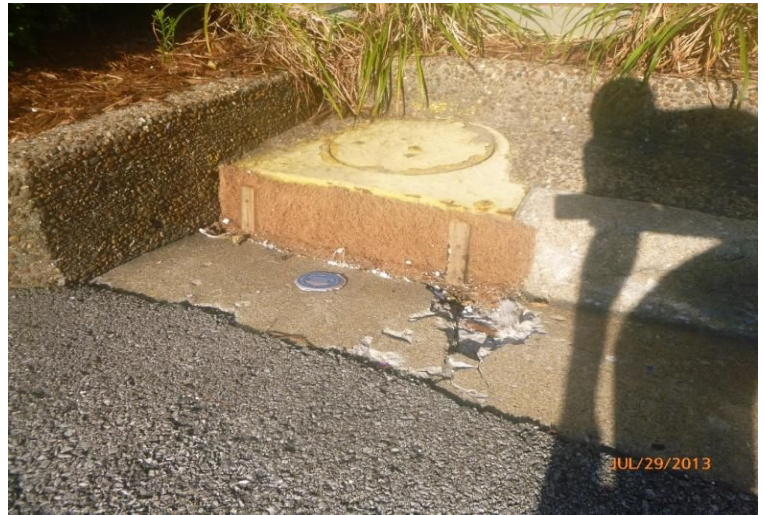
Do not remove manhole covers
